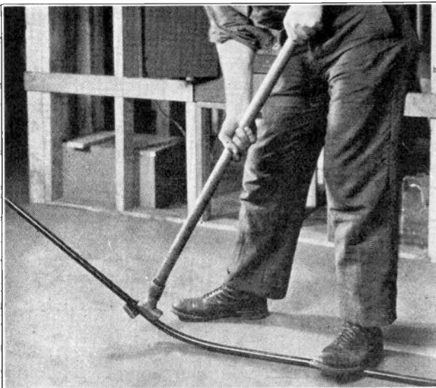
Fig. 63. Smaller sizes of conduit can be easily bent into the required curves and shapes with a bending "hickey", in the manner shown here.
