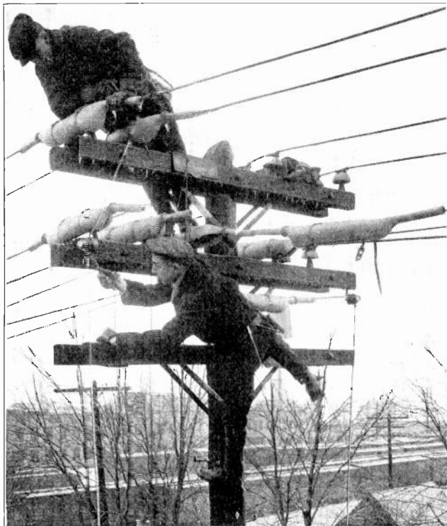
Fig. 368. This photograph shows the use of rubber line hose or "pigs" to protect linemen when working on live transmission or distribution lines. Photo Courtesy Lineman Protector Company.
