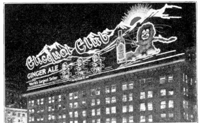
Fig. 208. Large signs of the above type often use several flashers, and a combination of lamps and Neon tubes to produce very beautiful effects.
