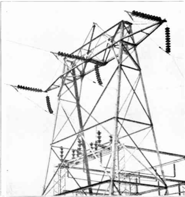
Fig. 343. This photo shows a heavy strain tower with strain insulators supporting the tension of the conductor span, suspension insulators supporting the conductor loops which run down to a substation, and pedestal type insulators in the background supporting high-voltage air break switches. (Courtesy Ohio Brass Co.)
