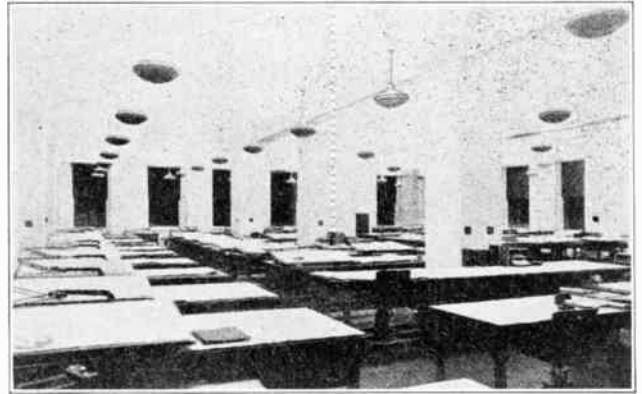
Fig. 182. This drafting room is lighted with indirect fixtures which throw their light to the ceiling first. The ceiling then reflects it downward to the working surface.
