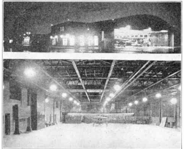
Fig. 233. The top view shows the outside appearance of a well lighted hangar, and below is shown the inside of the hangar and the arrangement of the lighting units.
