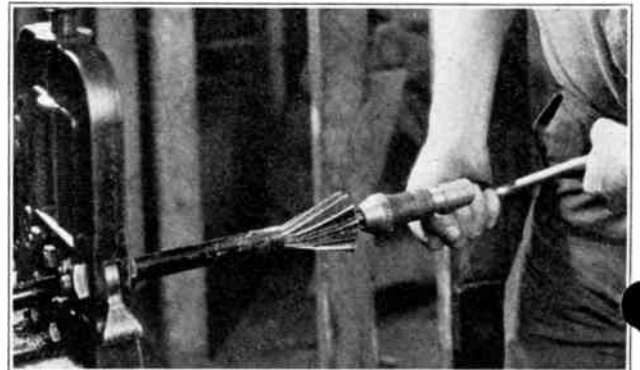
Fig. 61. Reaming the end of a piece of conduit after cutting to remove sharp edges, which might damage the insulation on the wire.
