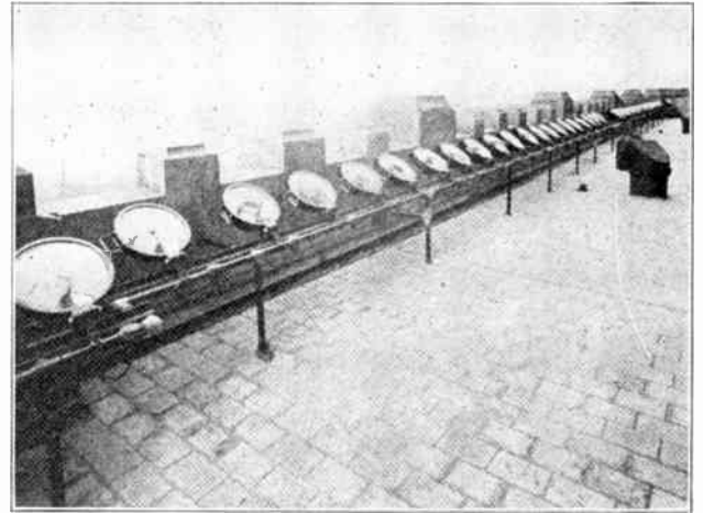
Fig. 214. This photo shows a row of flood light projectors in use on the top of a skyscraper office building. (Photo Courtesy Light Magazine).
