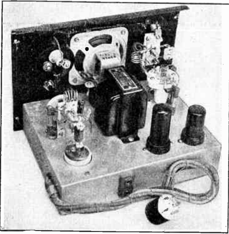
Fig. 1730 — Plan view of the transmitter-receiver. The acorn detector assembly is at the right, the transmitter oscillator at the left, and the audio equipment at the center.
