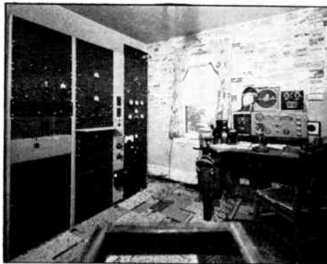
A high-powered station in a room with enough space to locate the transmitters along one wall and the operating table along another. Note the convenient location of the control switches, and the receiver raised above the table. (WICH, Worcester, Mass.)
