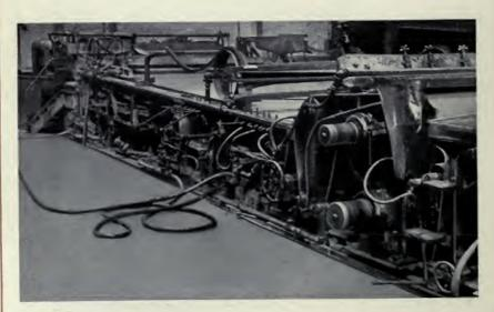
Where wood pulp is turned into Tribune newsprint. Wood pulp greatly diluted with water flows on a wire screen at the left of this picture. When it reaches the right end the water has been drained out, the fibres matted; it has become a sheet of wet paper—ready to pass through the series of rolls, blankets and driers, which finish the process.
