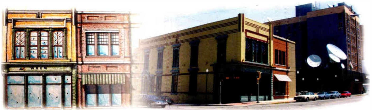
The QNI Broadcast Group Operations Center showcase Studio H and the renovation of the WGEM campus are great additions to Quincy's central business district.
