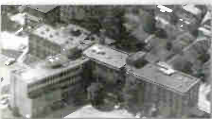
1960: Final Levering large addition and renovation completed making it a 150 patient hospital
