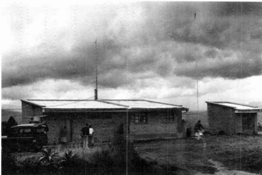
Radio Bahá'í AM transmitter at Cajas, Ecuador. The antenna mast is made from locally-available aluminum irrigation piping.
