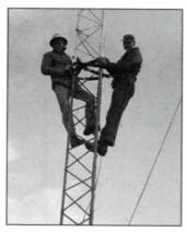
Bill Hartman and Ralph Fondell assembled the 250-foot tower in 10-foot sections.
