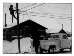
When the tower was assembled, Howie Nelson and Ralph Fondell strung cable from the studio to the transmitter site.
