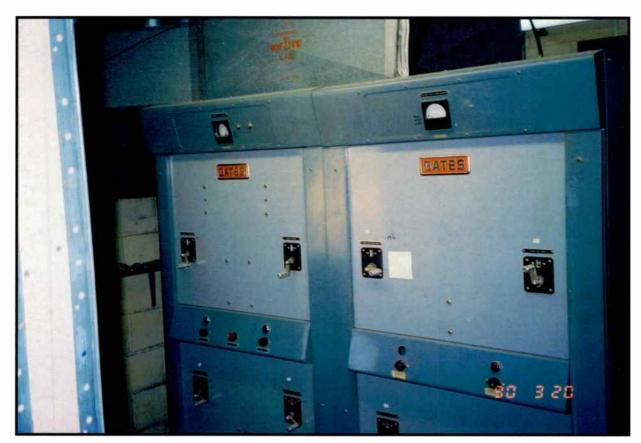
View of the KWNS AM Phasor banks, left is the daytime bank and the right is the nighttime bank. Normal antenna was 10.2 Amperes for the daytime pattern and 3.2 for the nighttime pattern. Just above the banks, the exhaust ductwork for the original Gates AM transmitter is still visible. The original Gates Phasor units are still in use today and with the four AM towers in back are all that remains of the equipment that Bill Huffman started the station with. This picture was taken in December 2007.
