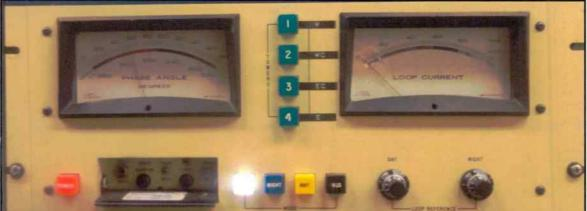
Potomac Instruments, Inc. Phase Angle Monitor, serial number 733 installed by Tim Hawks and Ron Detwiler in July 1975. The reason for replacing the original Gates monitor is lost to time. The FCC approved the new monitor and new readings on July 21, 1975. The monitor has been in continuous use since that time and has never been sent in repair, only recalibrated from time to time.
