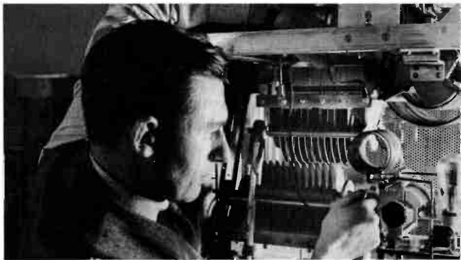
Placing a clip lead on the control apparatus.
