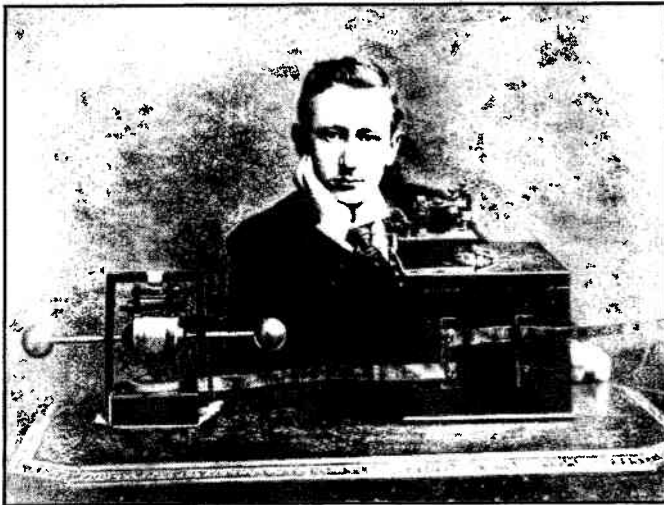
fig. 8 . The young Guglielmo Marconi photographed in London shortly after his arrival in February 1896. In front of him on the desk is the wireless apparatus he brought over from Italy. A Righi oscillator (part of the transmitter) is on the left, while on the right, a Morse sounder sits on top of a wooden box which contained a self-tapping coherer and a relay, making up the receiver. On the front of the box are two copper strips which acted as the receiving aerial.
