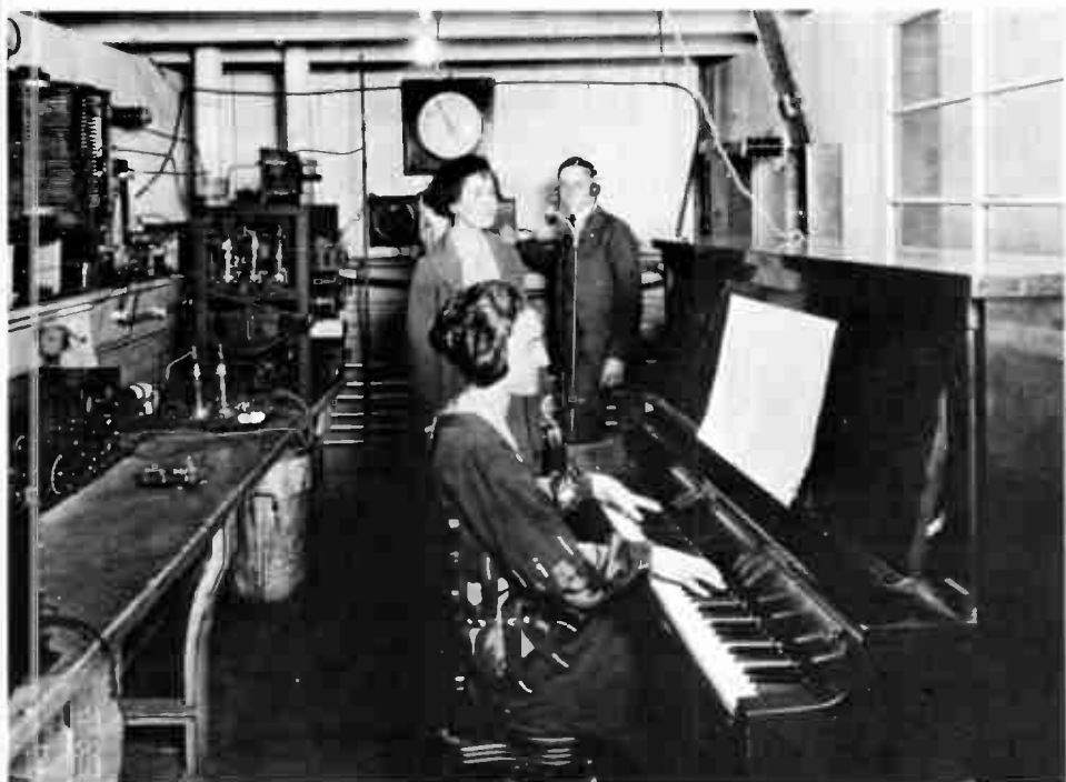
WBZ's station and studio occupied somewhat crowded quarters when started by Westinghouse at Springfield, Mass., in 1921.
