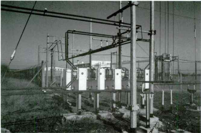
Figure 29.5 Antenna switch gear at Radio Monte Carlo
