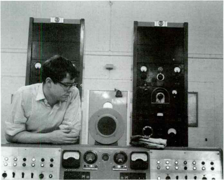
Figure 14.6 The original RCA transmitter control unit at Woofferton. Programme keys modulation meters in the centre of the desk with General Electric noise distortion and measuring equipment behind. Note the gloves for wave-changing on top of the desk
