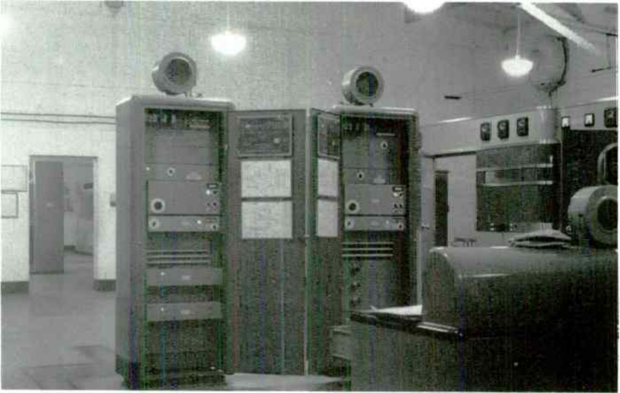
Figure 14.1 The Woofferton VOA relay station, England. 1944 RCA transmitters and programme input racks. Note the old-fashioned 'dalek' monitor loudspeakers
