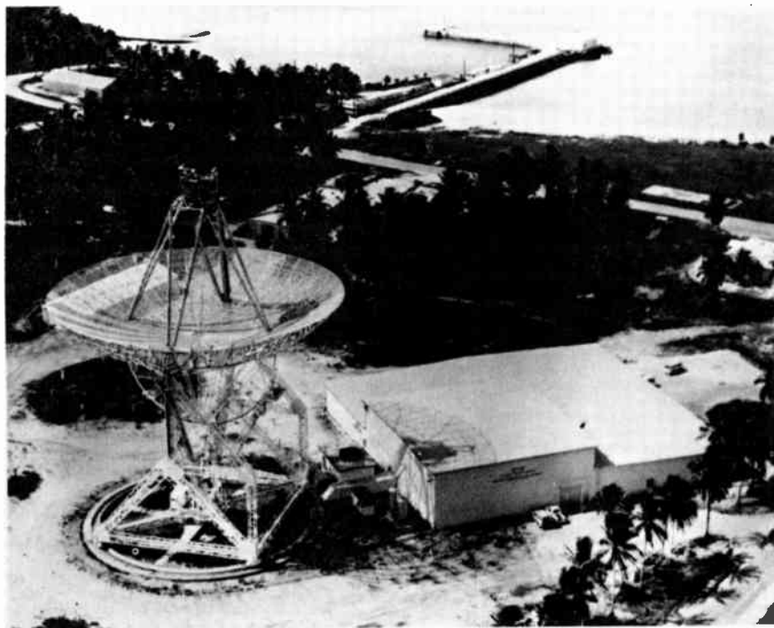
Fig. 63. The 150-foot-diameter parabolic antenna that tracks missiles on the Kwajalein Missile Range. Courtesy of General Telephone and Electronics Corp.
