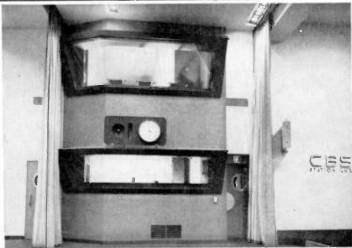
Looking forward into the control booth of a small studio. Notice the mike and the speaker on the board with the clock. This mike and speaker are the director's talk-back through which he directs the program.
