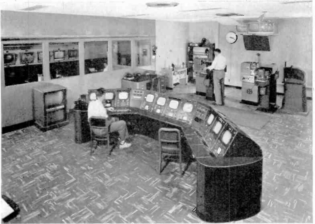
Design and construction of WHIO building and studios by The Austin Company
