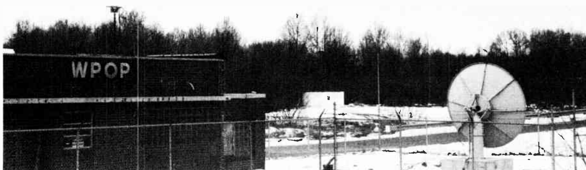
Fig. 15-1. Transmitter site. Many radio stations have studios in a central location, while the transmitter building and tower are out in the country. The satellite receiving dish (lower right) picks up network broadcasts that are relayed back to the studio. (WPOP-AM, Hartford, CT)
