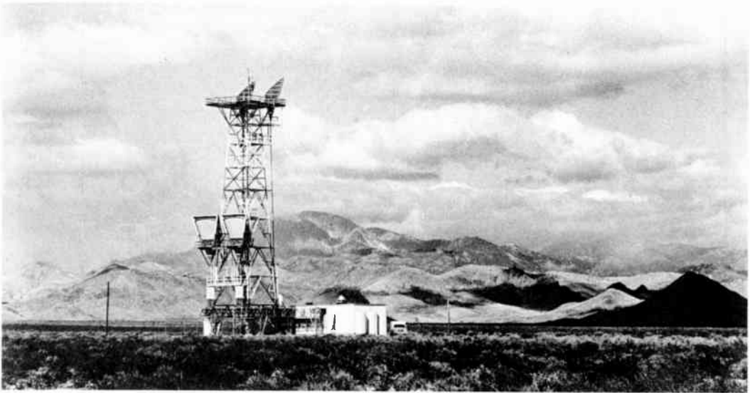
Figure 12-5 Microwave relay permits long distance communication without the use of cables. (AT&T)
