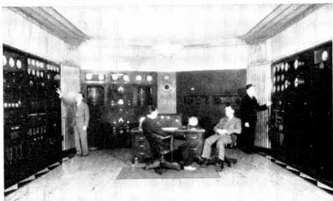
FIG. 22.—The transmitter room at WJZ, supervised by engineers and operators usually licensed for phone and code stations.
