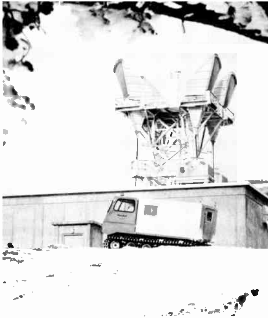
Exhibit 4.5 Microwave relay station
