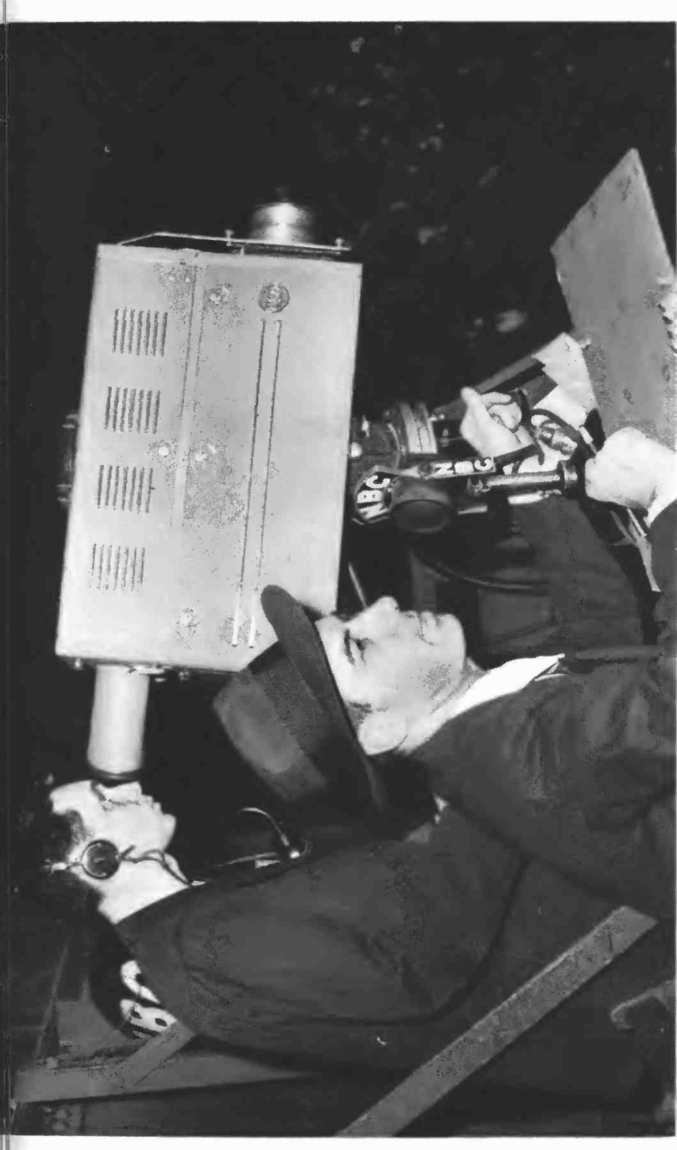
The television cameraman, looking through a viewfinder, adjusts the lens on the front of the camera which focuses the scene on the image orthicon, or electronic 'eye.' Bill Stern, sports announcer in the foreground, describes the game play-by-play.
