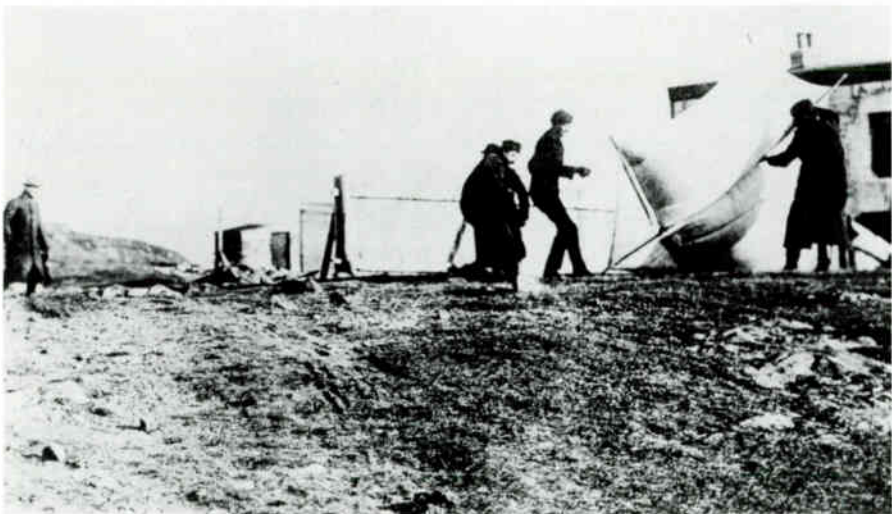
Marconi (on far left) observes as assistants raise the kite aerial used in detecting the first trans-Atlantic wireless signal on December 12, 1901. Marconi Co. photo.
