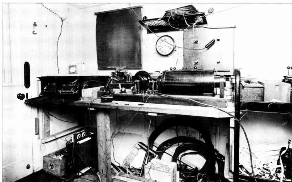
Marconi's wireless cabin on board the SS Philadelphia, February 1902
