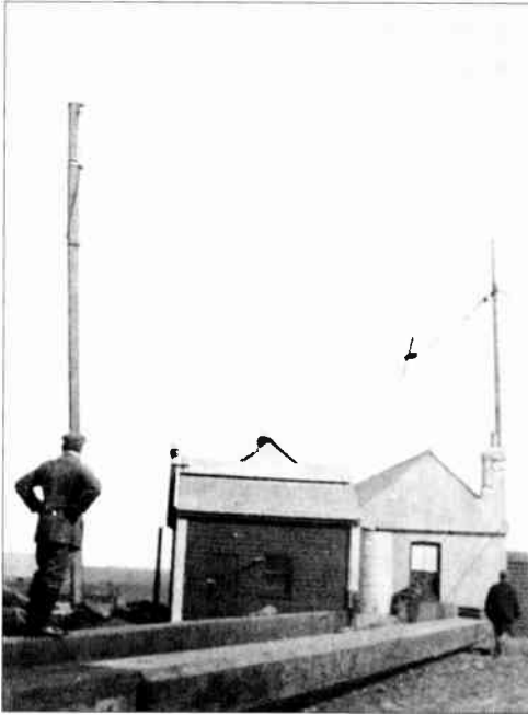
Poldhu site, April 1901. The first lowermast is on the left, erected with the aid of the derrick seen on the right
