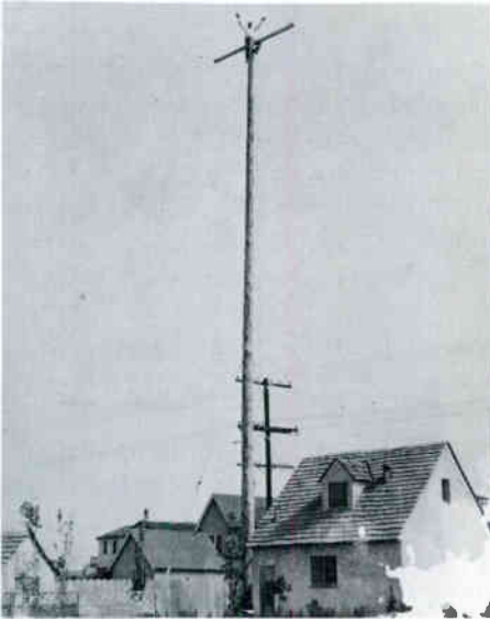
Don working on the rear pole, by the garage.
