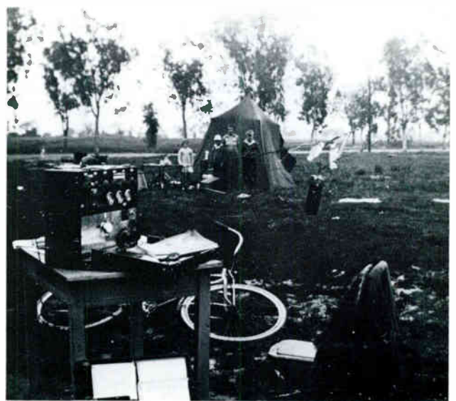
Don's portable transmitter set up in the field after the 1933 earthquake. Don's family stayed in the tent in the background.
