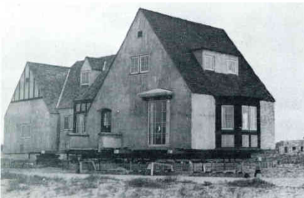
Doc Stuart's house was jacked up and moved in 24 hours.
