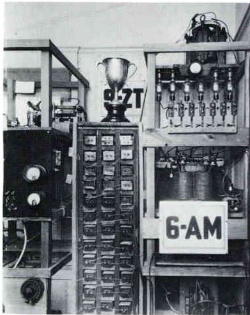
The 3-phase power supply at W6AM.
