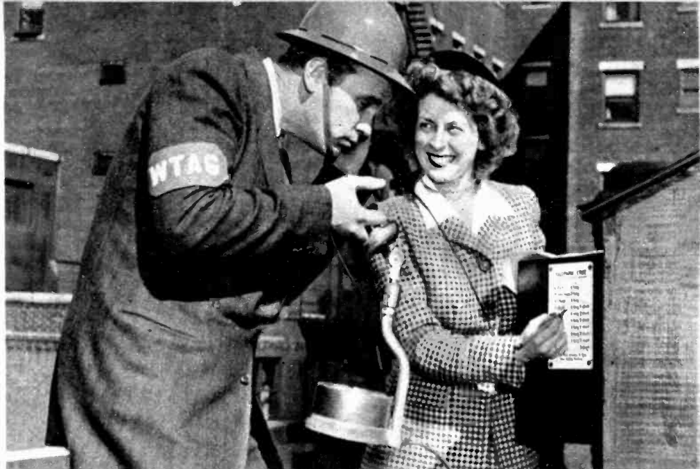
BOB DIXON AND MADELEINE SOHLSTROM TEST SIGNALS AND TELEPHONE COMMUNICATIONS.
