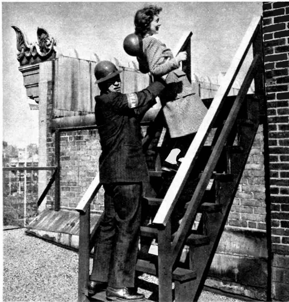
ONE OF THE STAIRWAYS WHICH CONNECTS VARYING ROOF LEVELS IN THE DEFENSE AREA.
