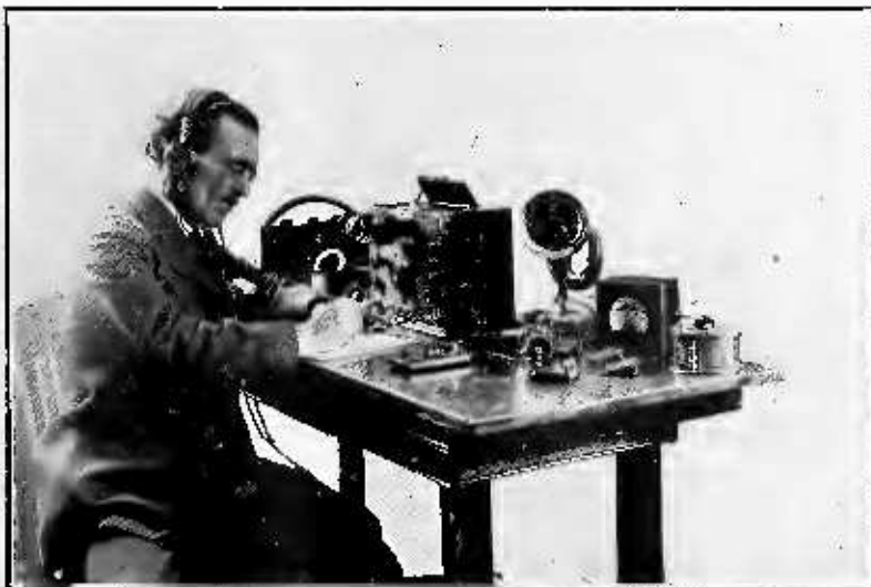
Engineer Milton Stilwell of the Areco Co.
