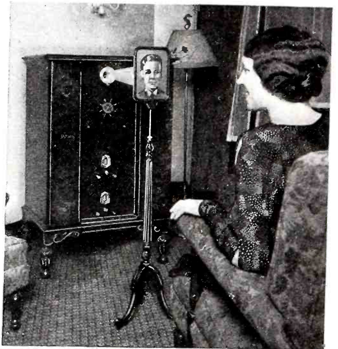
General view of the television transmitter used at W9XAP, showing the large group of photo-cells employed to "pick up" the image.
