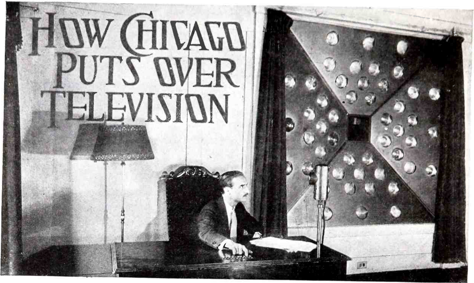
General view of the television transmitter used at W9XAP, showing the large group of photo-cells employed to "pick up" the image.
