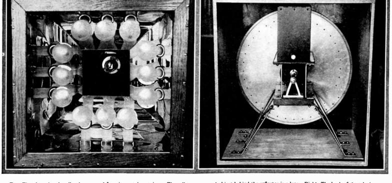
Top: The photoelectric-cell unit, removed from its metal container. The cell itself is the pear-shaped bulb in the foreground, the other tubes being A.F. amplifiers. Left: What you would look at if you were being "televised." The round object behind the reflector is a lens. Right: The back of the televisor, showing the photoelectric cell's can behind the revolving disc. The driving motor (not shown) fits on the baseboard.
