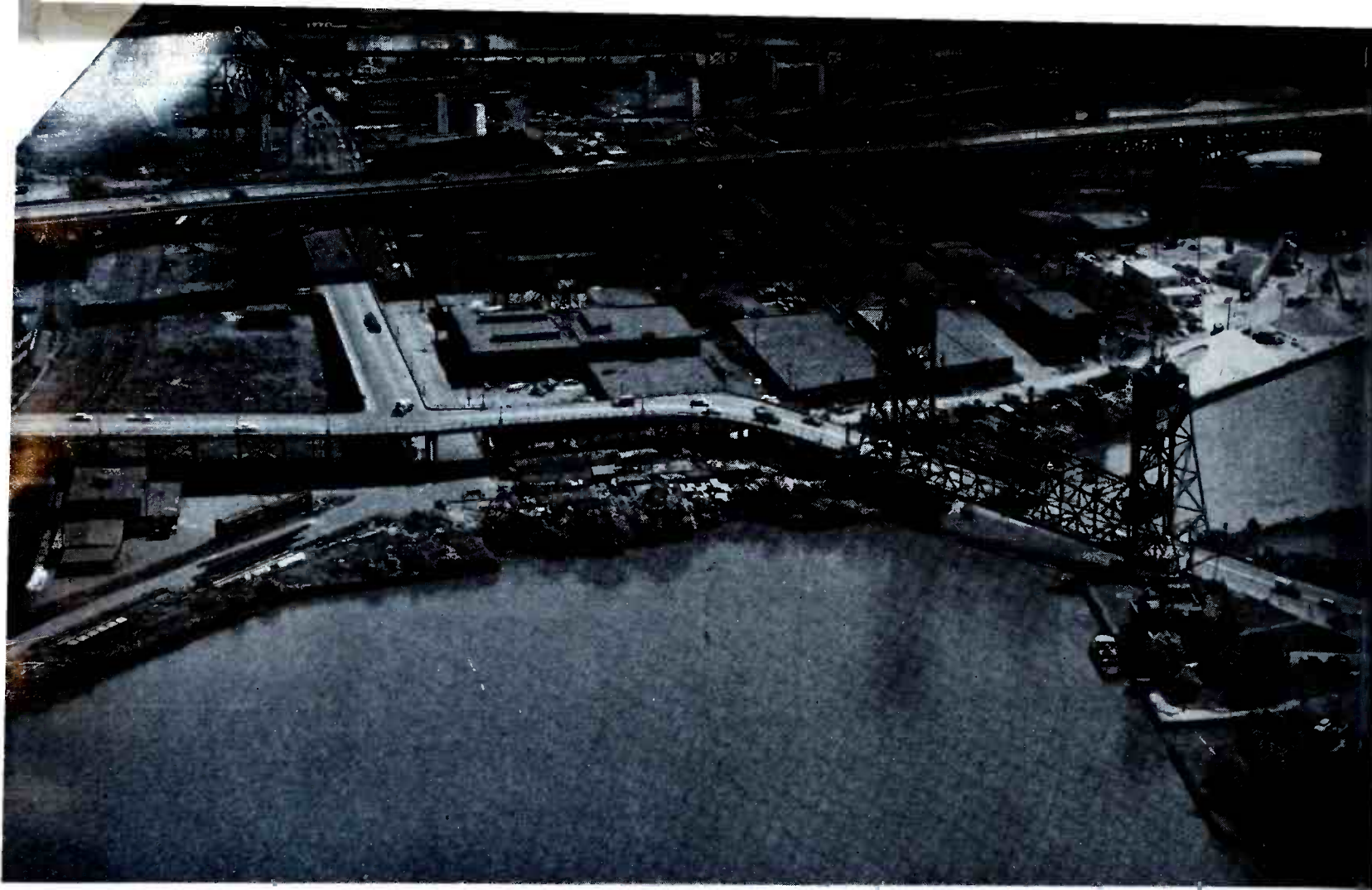
Typical of Cleveland's economic character is this photo of the Cuyahoga River showing industrial plants, fast modern highways, river transportation, and railroads.
