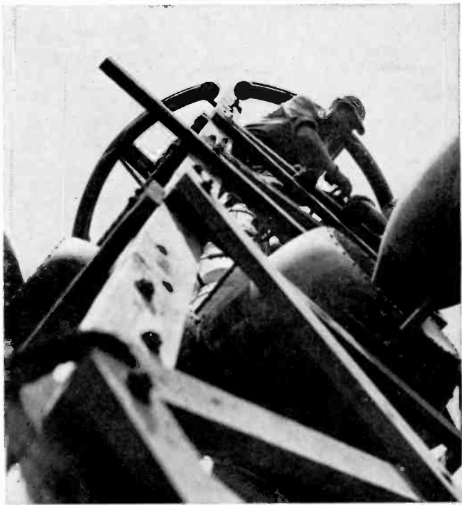
Steeplejacks at work on an NBC television antenna—1250 feet above the sidewalks of New York. Its height gives telecasts a wider range in the New York and New Jersey area.
