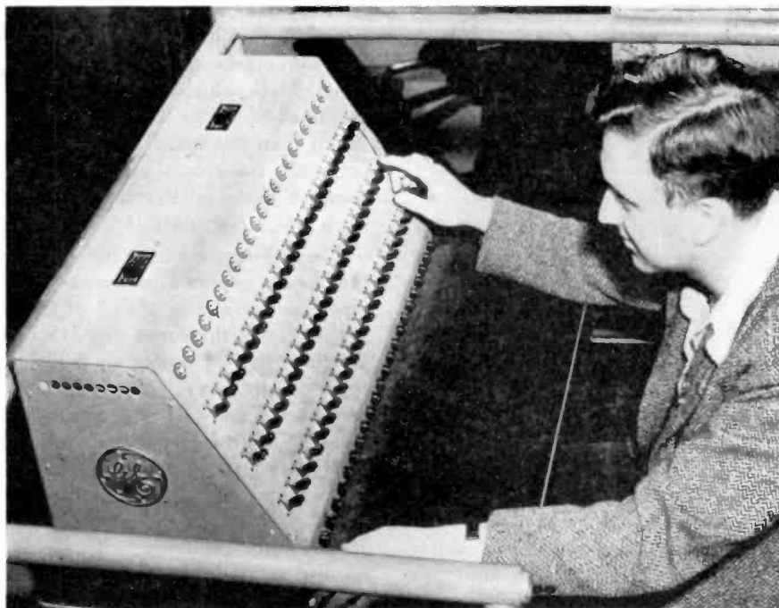
Lighting console which makes possible individual operation of the various circuits
