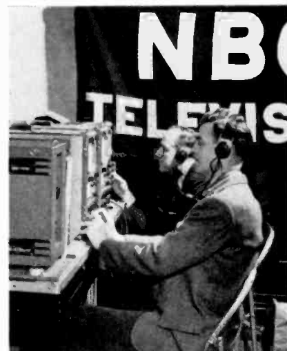
Control room in Garden
