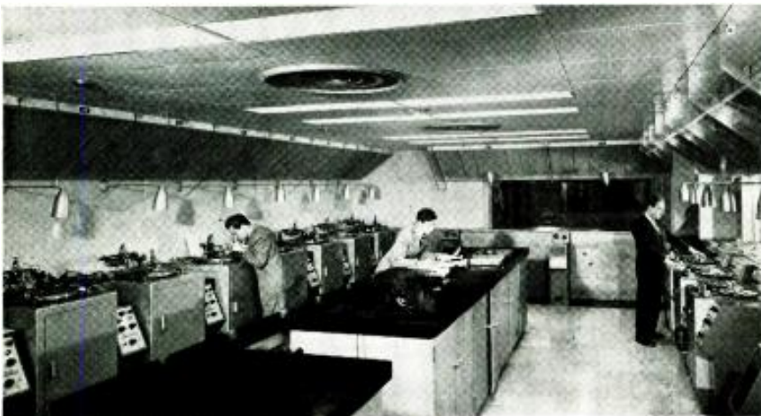
Recording room in new thirteen-floor Radio Canada building in Montreal, where any of 50 programs passing through master control can be chosen automatically for recording. Each of fourteen recorders (disc or tape) which has its own control panel, clock, light and overhead speaker, can record simultaneously or separately. The building, with 26 studios, will soon feature three special studios for TV. From these studios in a five-story television wing, CBC will produce TV programs for broadcast from a transmitter atop Mount Royal. The entire TV wing has been so constructed that two more floors can be added if necessary. All the television equipment for the three studios has been ordered. Standard video equipment has been ordered while the accompanying sound equipment is being manufactured in Canada to CBC design and specifications. CBC television in Montreal will also operate a mobile van for outside events (sports, etc.). The van will have its own transmitter and portable equipment.
