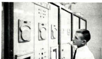
To energize the amplifiers, a new highly reliable 6000-volt d.c. shore-based power supply was developed. It sends precisely regulated current along the same coaxial conductors that carry the communication channels, despite varying earth potentials between the continents or islands on which the terminals are located.
