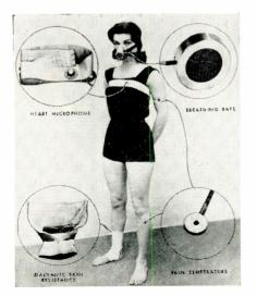
Fig. 6: The welldressed space pilot will wear many of the se medical instruments (designed by Gulton Industries, Inc.). The y will measure heart reactions, breathing, temperature, and resistance to shock and stimuli. The breathing rate apparatus, can even tell if he is alive or unconscious.
