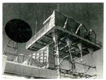
New high speed method of transmitting scientific and business data by microwave is now being used by North American Aviation, Inc. Dish at left on Oat Mountain receives microwave signals from Rocketdyne, 9 miles away, then beams them to Los Angeles 30 miles away.
