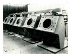
Airborne Tactical Data System consoles are set-up for preshipping tests.
