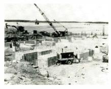
Power plant foundations. Five large blocks run at right angles to the length of the building. The two small blocks (left, foreground) are foundations for small generators.
