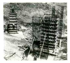
Tower foundation. Deep excavation was made through very soft grey marine clay to reach bed rock.
