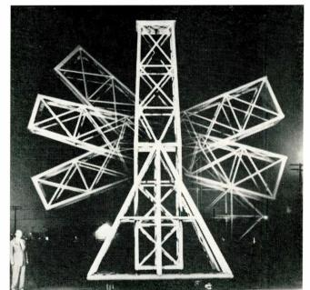
special high glass content reinforced plastic tubes, exceedingly strong and rigid and resembling a welded tubular steel structure in appearance. The use of fiberglass reinforced plastic tubes as primary and secondary structure assures virtually no pattern interference.
