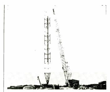
Erection of towers. The gin pole suspended in center of the tower is used at heights above 200 ft. to raise tower material for erection.
