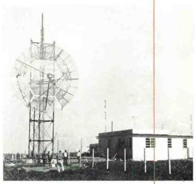
This 28-ft. parabolic antenna at Dorado, Puerto Rico, is part of Federal Telecommunication Labs 238-mile "over-the-horizon" nicrowave link to the Dominican Republic. The link operates on a 891 MC with a power of 500 watts.
