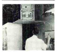
CLOSED-CIRCUIT TV is scanned in tote room by American Totalisor Co. engineer at Del Mar racctrack to be sure inside figures correspond with those on infield tote board. Equipment designed and made by Kay Lab.
