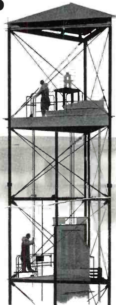
Long elevator ride takes men up to within 24 feet of top. They mount ladder for final ascent.
