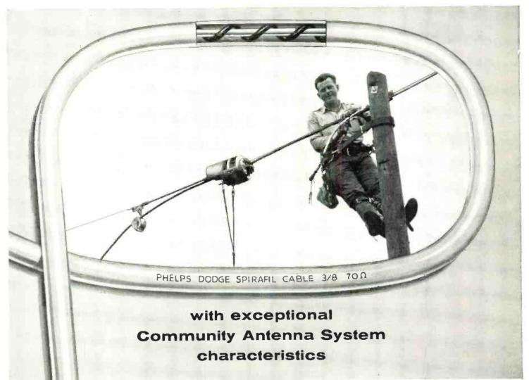
Spirafil coaxial cable was developed by Phelps Dodge as a companion cable to Styroflex coaxial cable. It is particularly adaptable to use in community antenna systems. For this purpose, it has a number of outstanding features—no radiation, low attenuation, excellent frequency response, uniform electrical properties over wide temperature variations and unlimited operating life.
