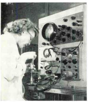
Presetting cavity resonant frequency.
