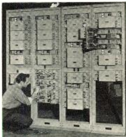
Multiplexing equipment gets final touches
