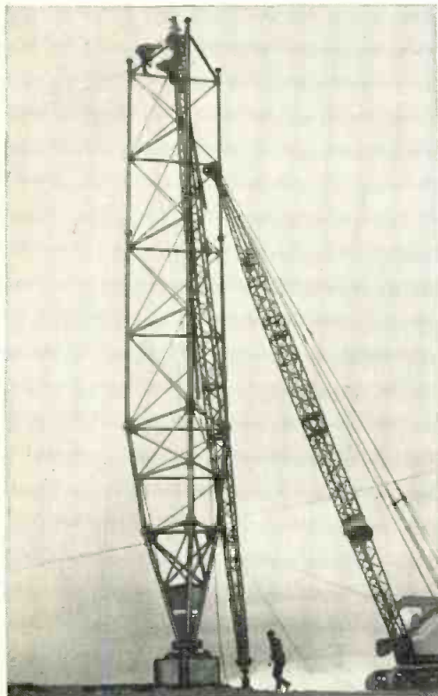
Construction close-up on new 1282-foot Truscon Triangular Guyed Tower for WWTV in Cadillac, Mich.
