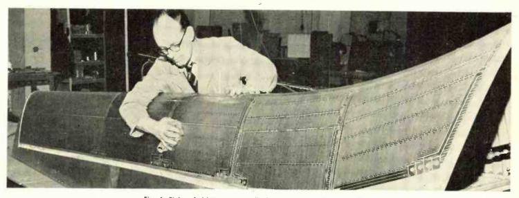
Fig. 4: Fixing de-icing mats to tail plane of Bristol Britannia airliner
