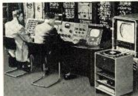
Fig. 18: Control console with color monitors
