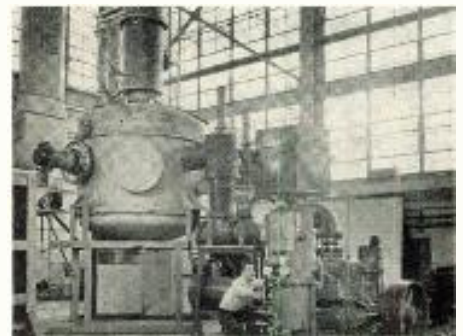
Undergoing final tests is the modular type 1000-pound high-vacuum furnace.
