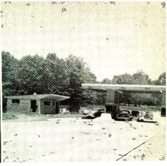
Fig. 6: Beckley toll booth. VHF equipment left
