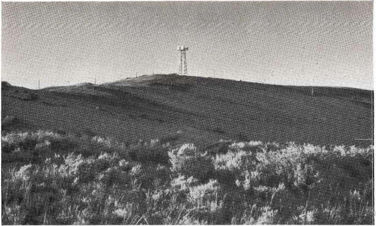
Radio-relay station at Evanston, Wyoming
