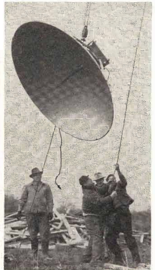
Fig. 8: Six-foot microwave dish at the start of the haul up the 150-foot Bordentown tower
