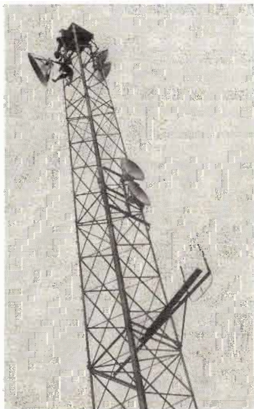
Fig. 1: Six-foot parabolic antenna nears top of 150-foot tower at Bordentown. Two microwave dishes halfway down the tower link network to police center at W. Trenton. VHF antennas at lower right contact outlying mobile stations
