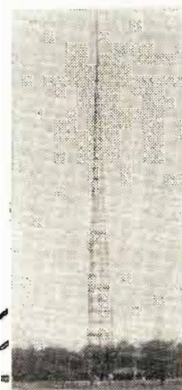
Truscon Type H-30 Self-Supporting Tower, operated by WEXL-FM, Detroit, Mich., supports an 8-bay General Electric F-M antenna and rises to an overall height of 425 feet.
