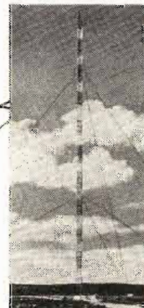
Truscon Guyed Radio Tower, WKY, Oklahoma City, Oklahoma, is 956 feet high to top of FM antenna.
