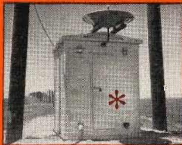
* This is one of the microwave equipment shelters on the Rock Island system. It holds the repeater unit and Onan generator.
