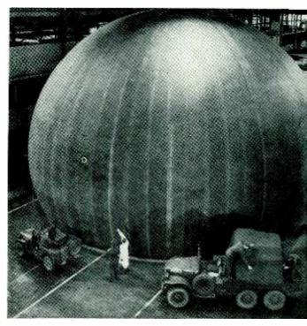
Rubberized fabric radome made by Firestone to protect Air Force radar installations from wind, snow, sleet and ice. Radome will be mounted atop a 25-foot tower. The balloon-like shelter, held up by a twentieth of a pound of air pressure, over all measures 167 feet in circumference and 36 feet in height. Inflated to half-pound pressure, the radome is designed to withstand 125-mile-an-hour winds. Deflated, it packs into a canvas bag like the one on Army truck in foreground.
