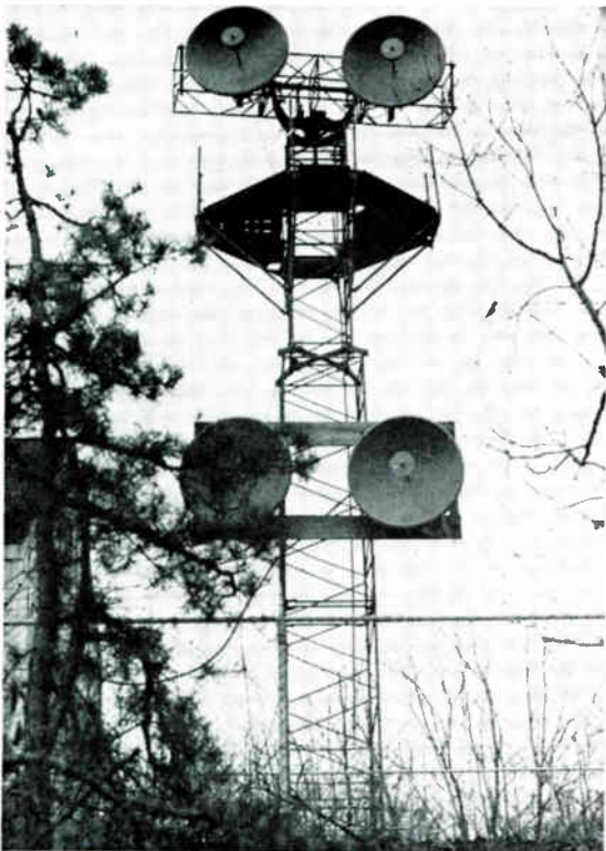
Fig. 1: (Below) Two complete CWTR-5A equipments that have been under continuous test operation. (Left) Antennas used with 952-960 MC installation
