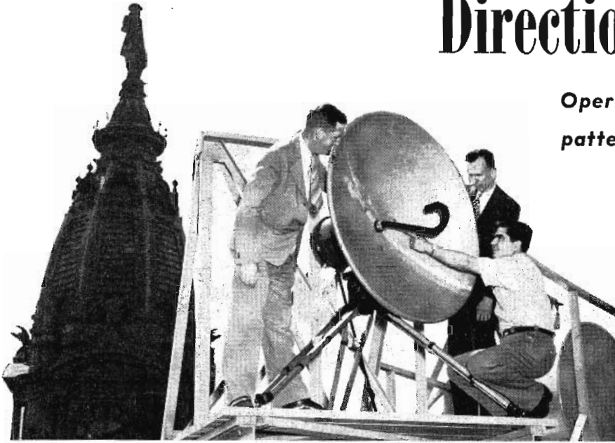
TV microwave relay equipment installed on the City Hall building in Philadelphia, Pa.
