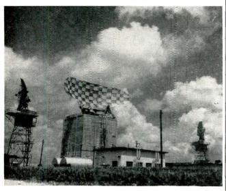
The Air Force's AN/FPS-35 shown at Thomasville Aircraft Control & Warning Site, Alabama. Sperry Gyroscope was system manager. Antenna weighs nearly 70 tons. Tower is 85 ft. high and 60 ft. wide.
